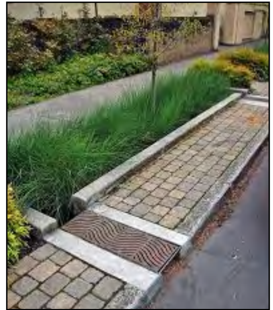
Roadside bioretention. Source: sitephocus.com
